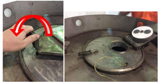
2. Take note of the gap between the male and female ends of the fusible link before removing the roll pin
